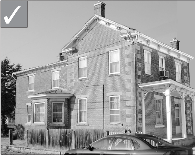
Preserve an older addition that has achieved historic significance in its own right as this one has. (Sainte Genevieve, MO)
