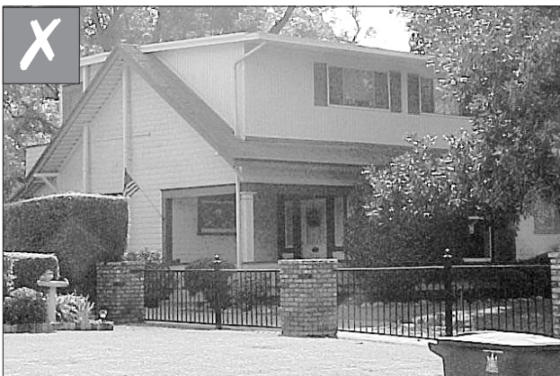
A new dormer should remain subordinate to the historic roof in size and character. The dormers on the front and rear of this structure are too large and are inappropriate. (Memphis, TN)
