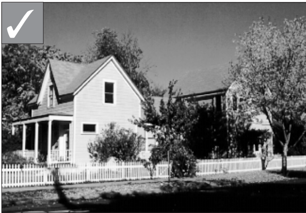
Design an addition to be compatible in size and scale to the main building. This addition appears to be in scale with the original building because it is separated with a smaller connecting structure. (Napa, CA)
