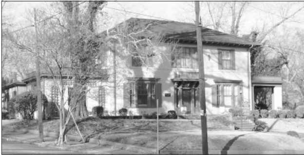
The first step in planning a preservation project is to identify any significant features and materials of the structure.
