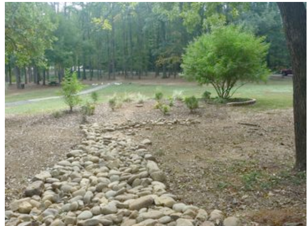
Rock bed intercepts stormwater and directs it to rain garden.
