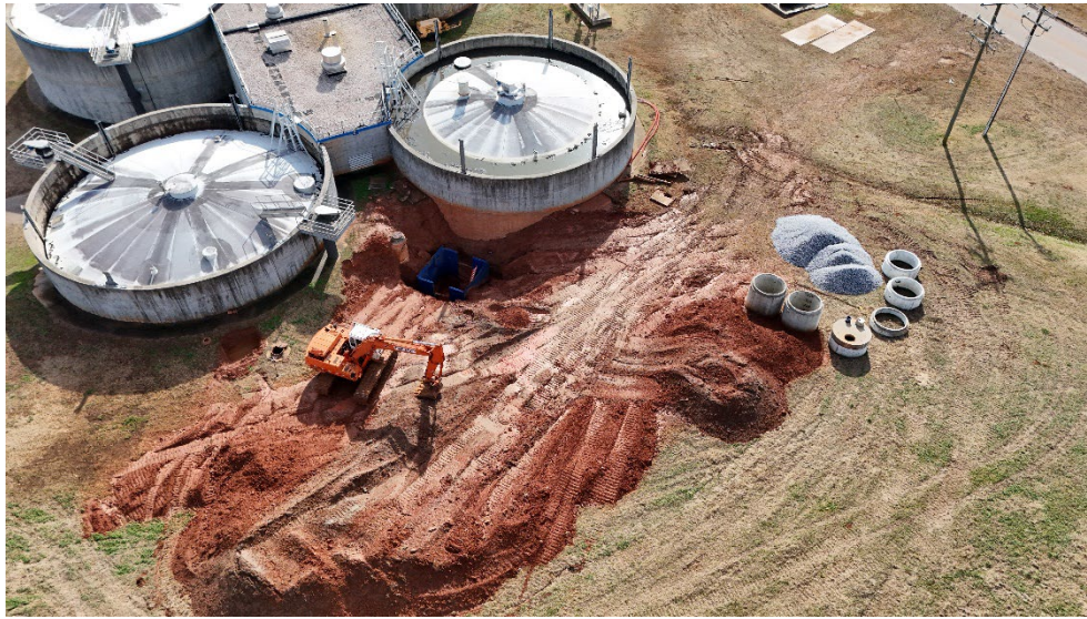
Aerial view of Digester Project at the Rocky River Plant
