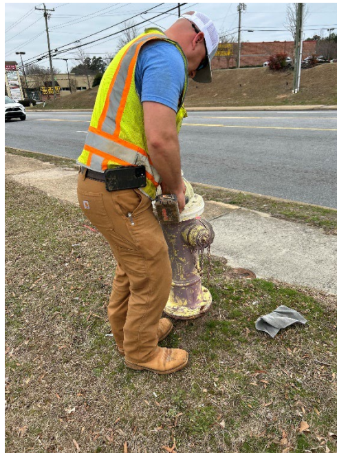
Water Department employee performing fire hydrant maintenance
