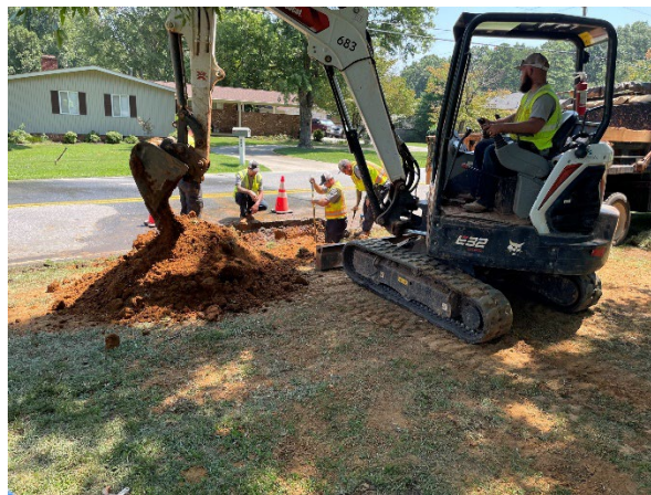
Water Ops crew at work
