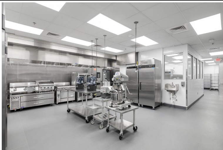
Completed kitchen inside Shared Kitchen
