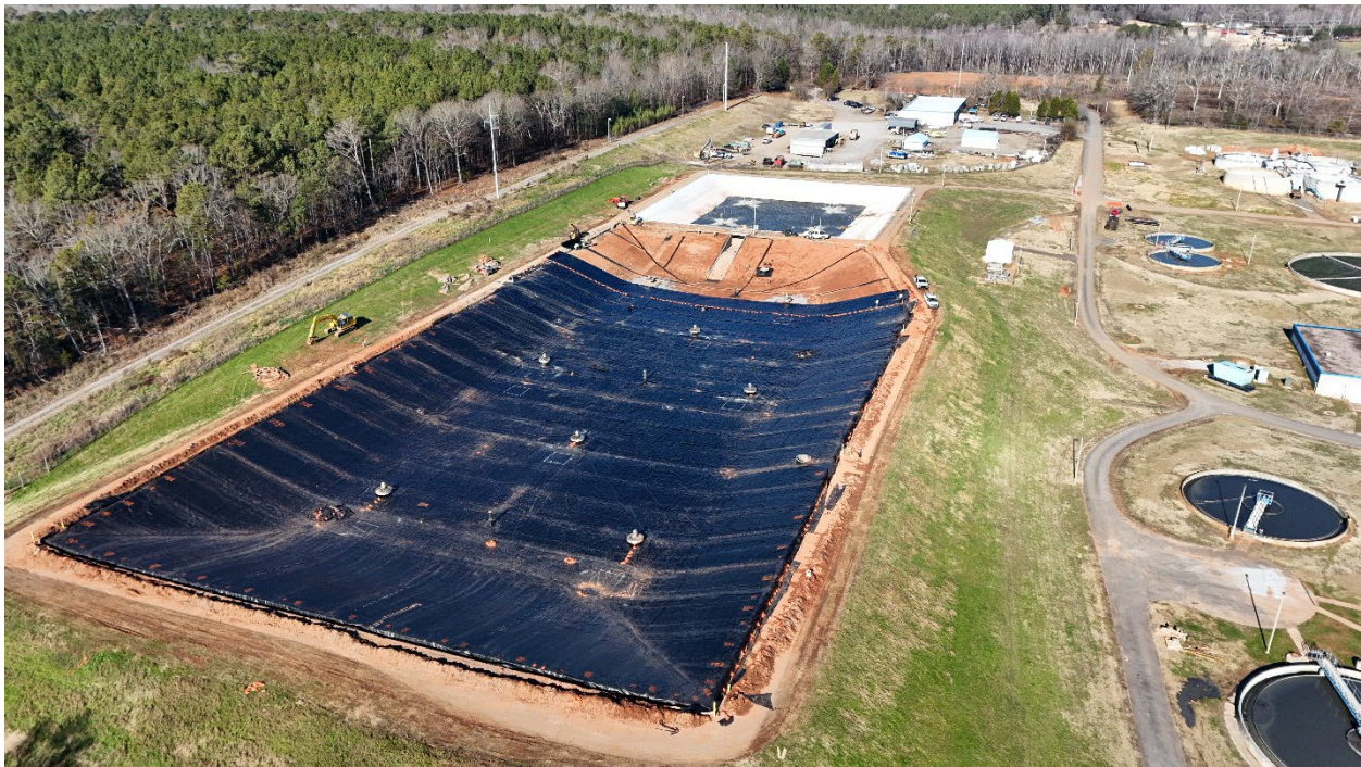
Aerial view of Rocky River Basin Liner Replacement project.
