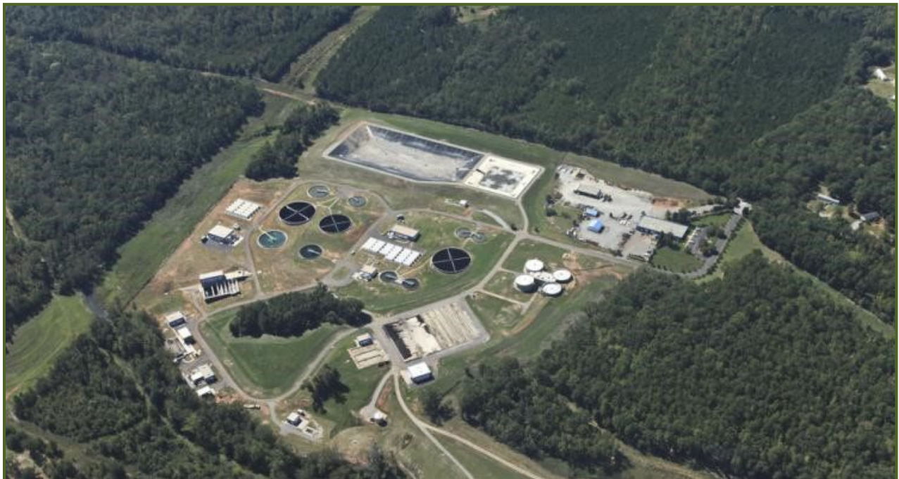
▼Rocky River Wastewater Treatment Plant Expansion Funded in part by 2009 Water & Sewer Revenue Bond
