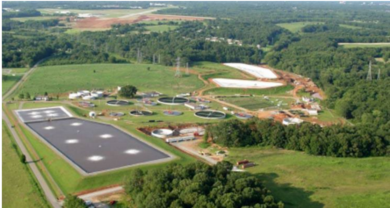
Generostee Treatment Plant
