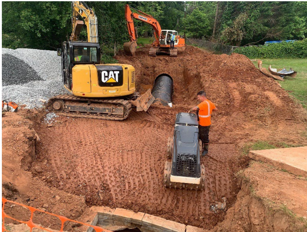
Construction on a Stormwater project
