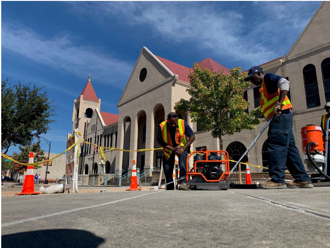
Street crew working on South Main Street Crosswalk
