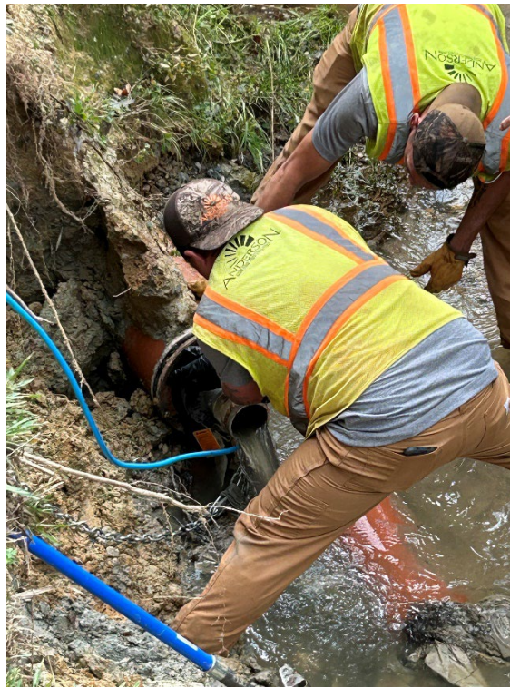
Sewer crew at work
