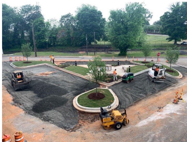
Public Works crews working on the Textile Point project
