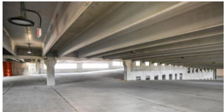
Interior floor of East Market St parking garage
