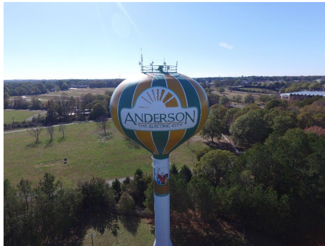
City of Anderson water tower
