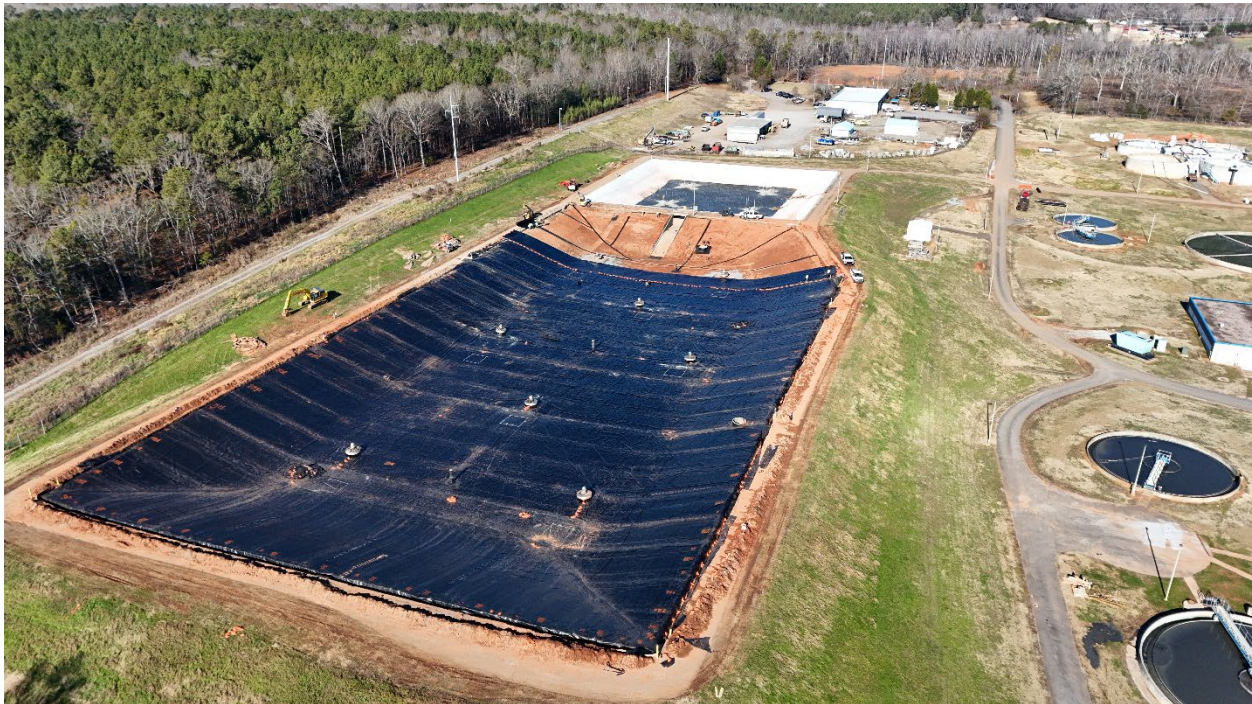
Aerial view of Rocky River Basin Liner Replacement project.
