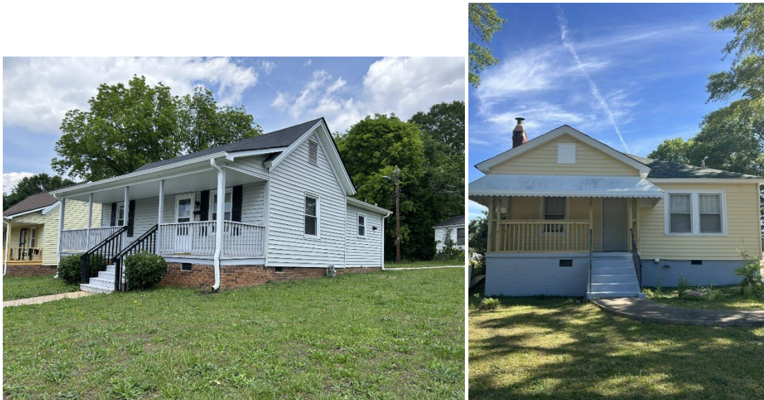
Completed exterior of rehabilitation projects
