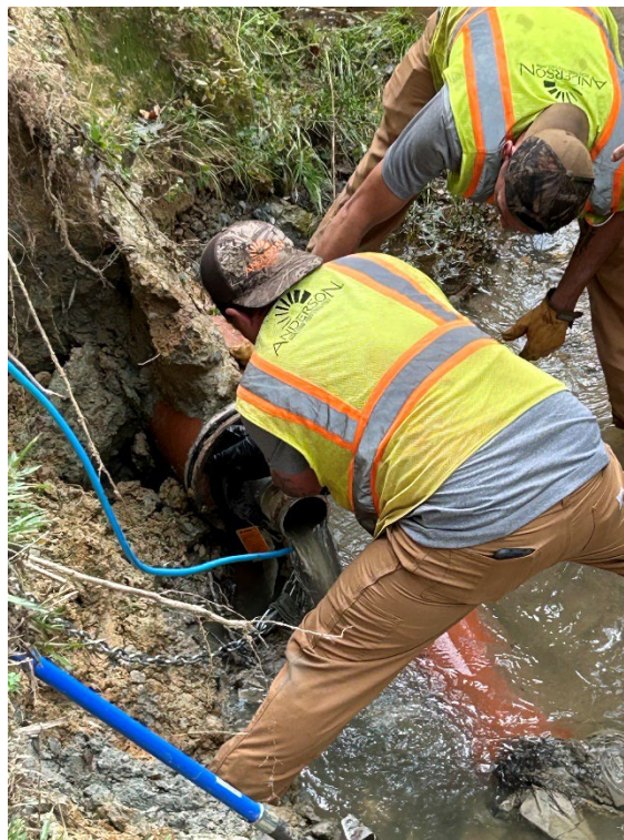
Sewer crew at work
