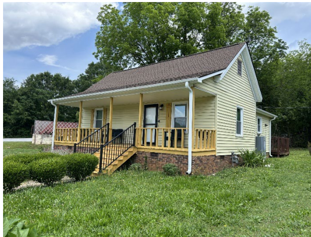
Completed exterior of rehabilitation project
