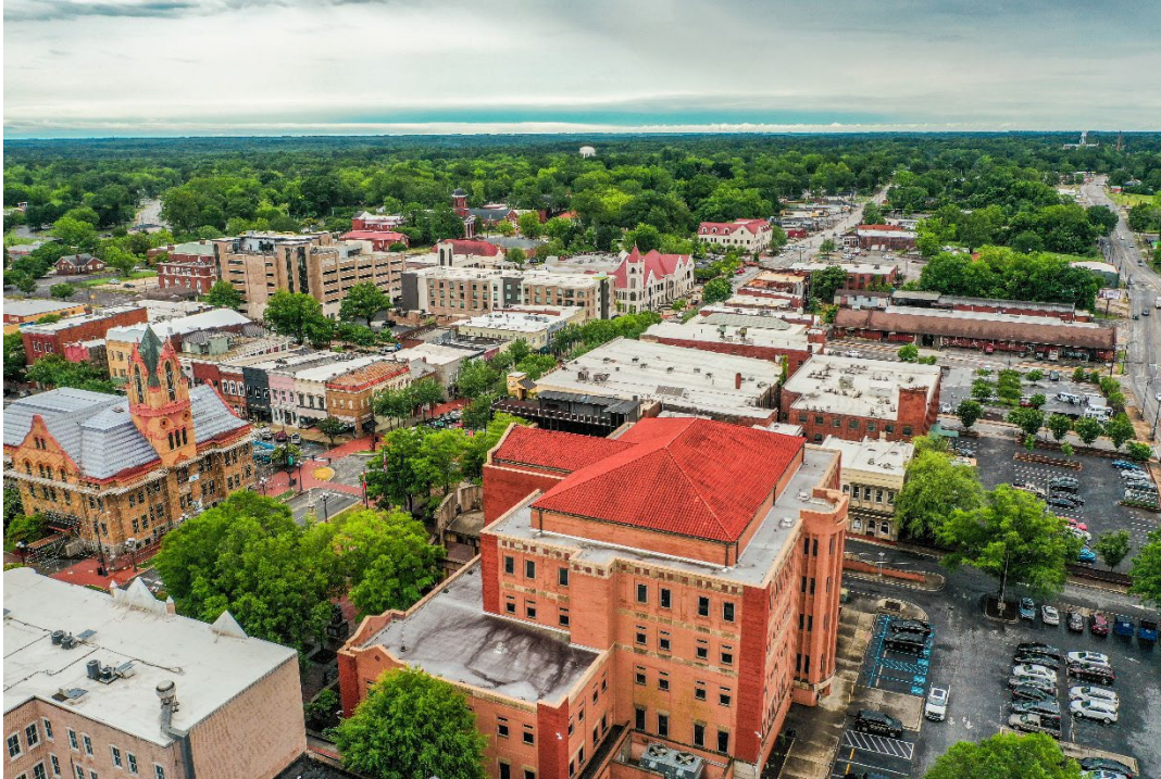
Aerial View of Downtown Anderson
