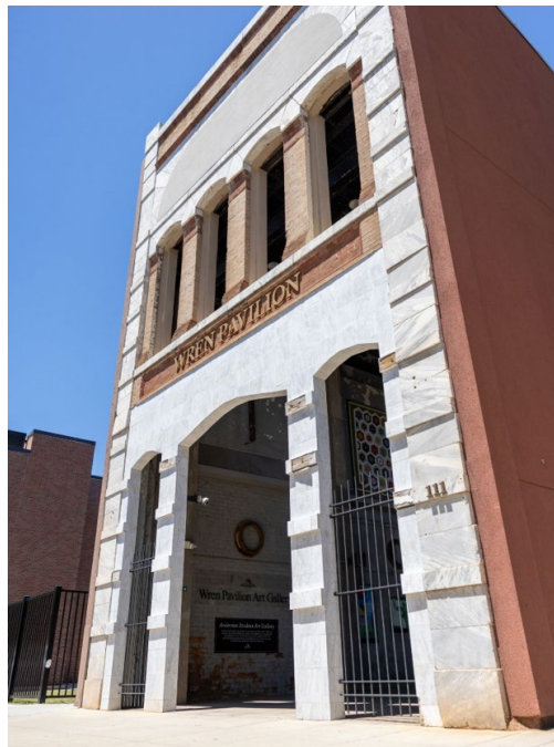
Entrance of Wren Pavillion
