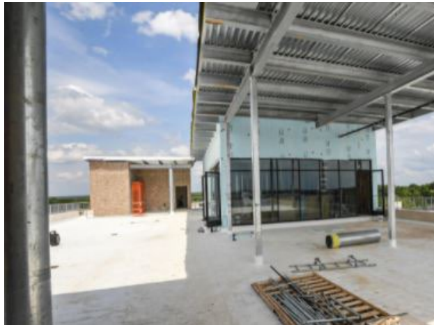
Rooftop construction of the East Market St parking garage prior to completion
