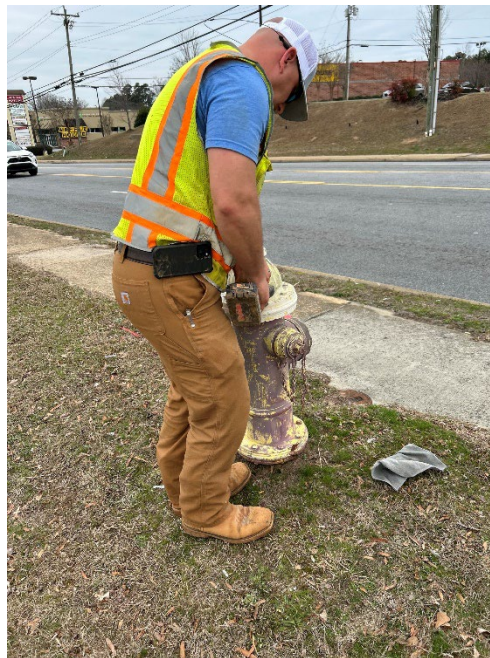
Water Department employee performing fire hydrant maintenance
